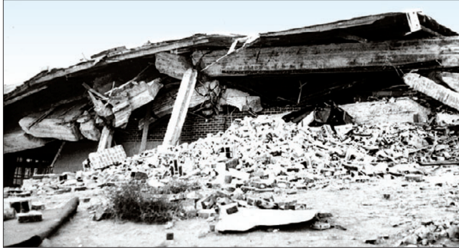
Figure 4-6: Collapse of portion of nonductile concrete frame school structure, Helena, MT, 1935
