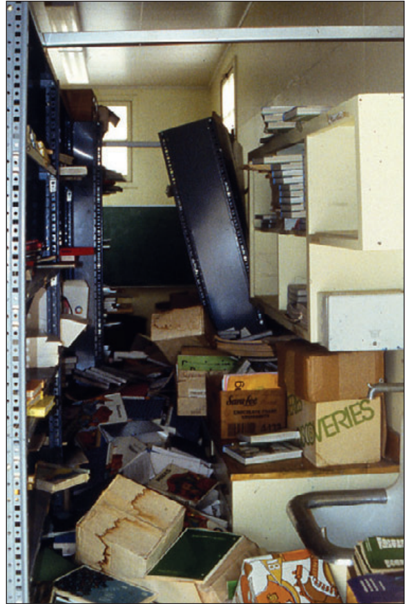
Figure 4-8: Fallen filing cabinets and shelves, Northridge, CA, 1994
