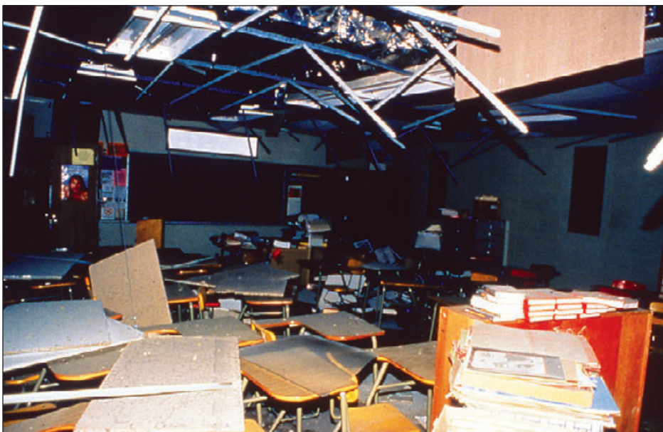
Figure 4-25: Ceiling damage, Northridge, CA, 1994
