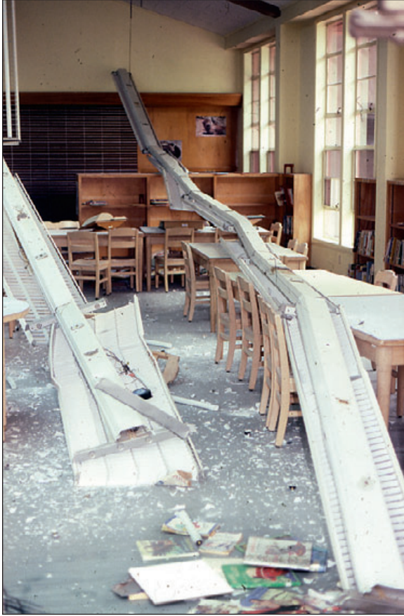
Figure 4-10: Fallen light fixtures, library, Coalinga, CA, 1983
